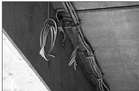
X-ECH for fastening bunched cables
